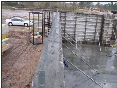
A cast-in-place concrete wall just after pouring and placement of truss tie-down embeds.
