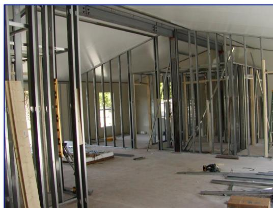
Home Front, Inc. uses a steel moment frame to improve wind resistance and steel studs to increase termite resistance. (Source: Home Front, Inc.)
