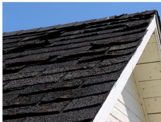
Loose/Brittle Shingles
